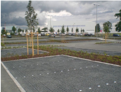
Permeable surface treatment within planted parking areas
