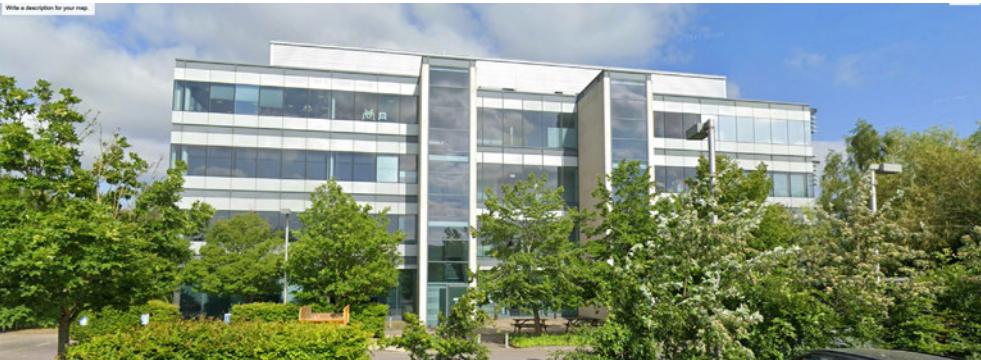
Office element, Green Park, Reading
