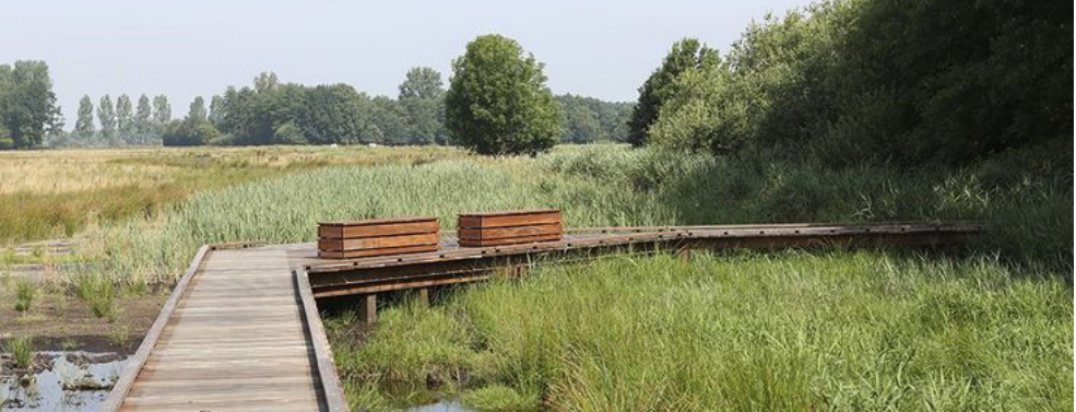
Routes and paths: hardwood forest trackway footbridge, Bergen, Netherlands
