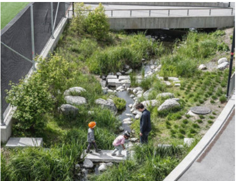
SuDS integrated between the service area and road
