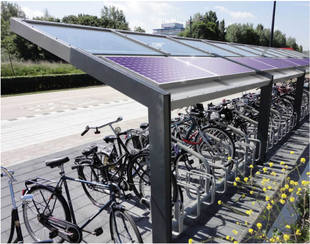
Solar PV panel cycle roof, Netherlands
