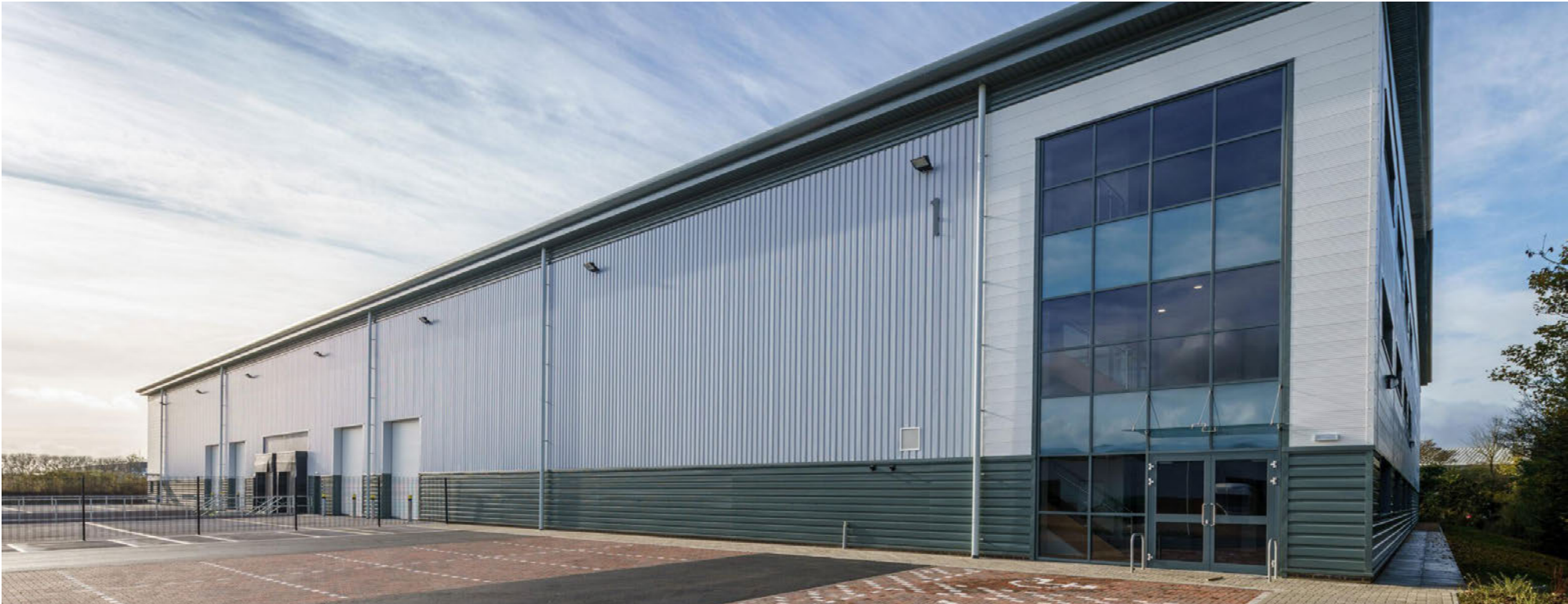
Industrial steel material, Gateway 12 Business Park, Gloucester
