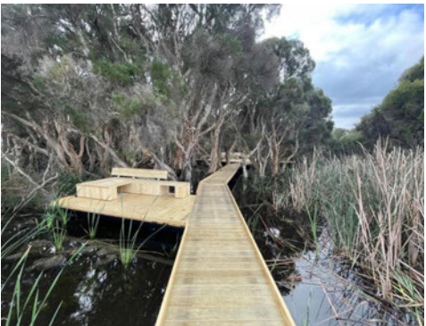
Timber wetland boardwalk
