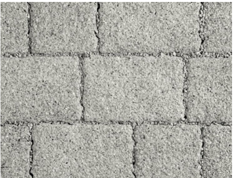
Permeable block paving
