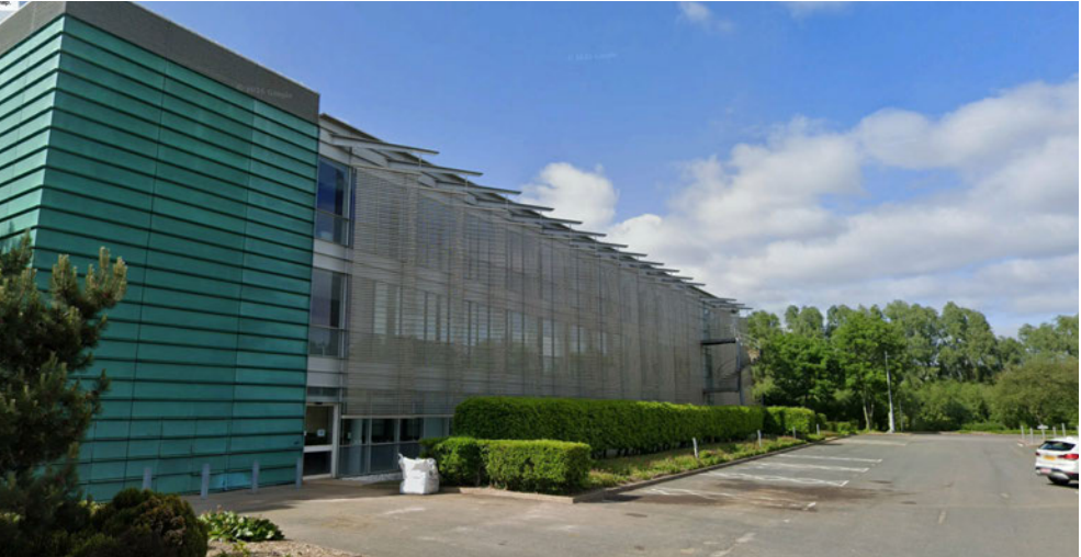
External solar shading, Green Park, Reading
