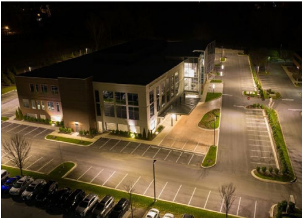
LED light car park, North Carolina
