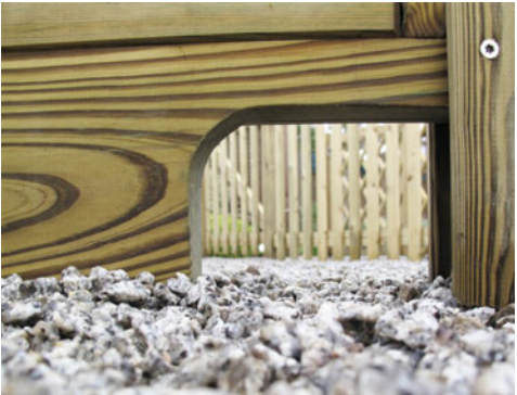
Hedgehog access integrated within the fence and gravel-board system
