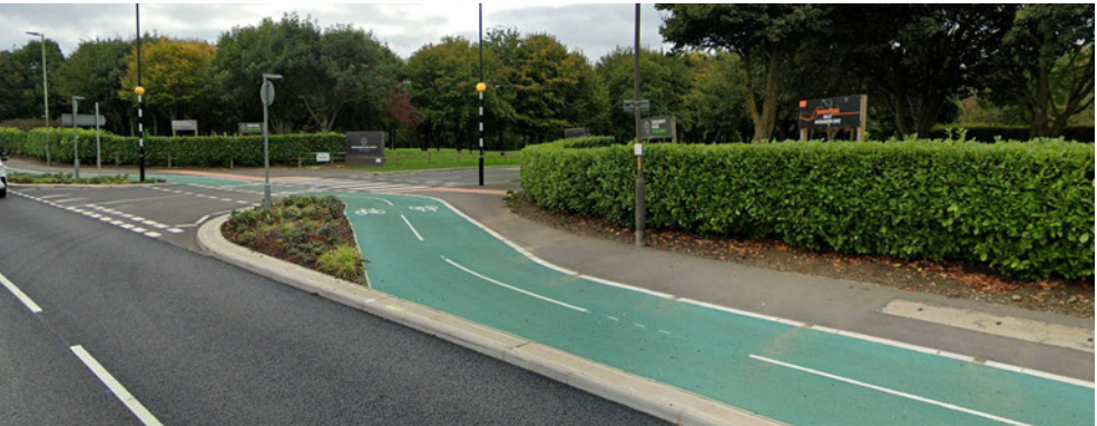
Segregated cycle lane and crossing, Meteor Business Park, Gloucester
