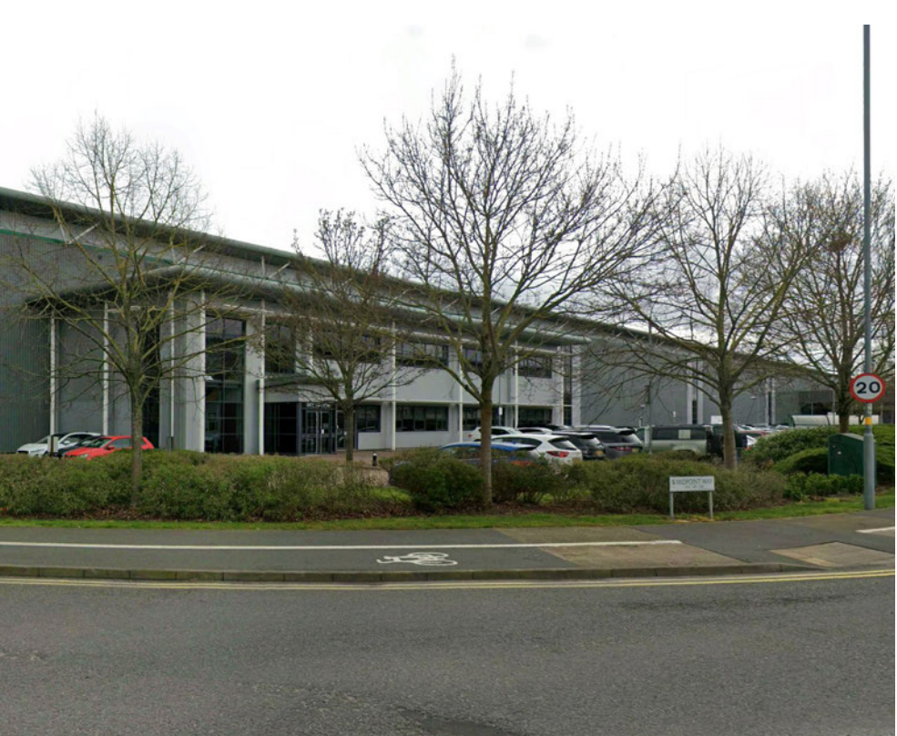
Entrance creates visual break, Peddimore industrial Estate, Sutton Coldfield, Birmingham
